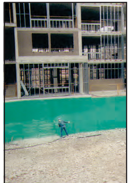
Above: Rub-R-Wall applied over poured concrete surface of foundation walls.
