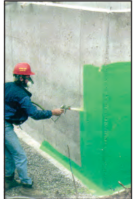
Above: Rub-R-Wall applied with pressure spray.
