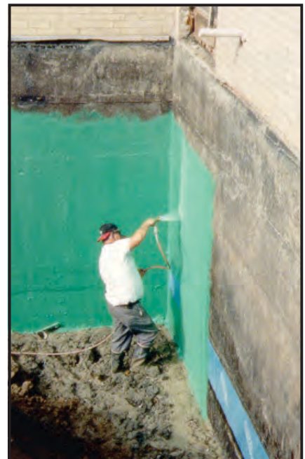
Above: Rub-R-Wall installed in retrofit application.
